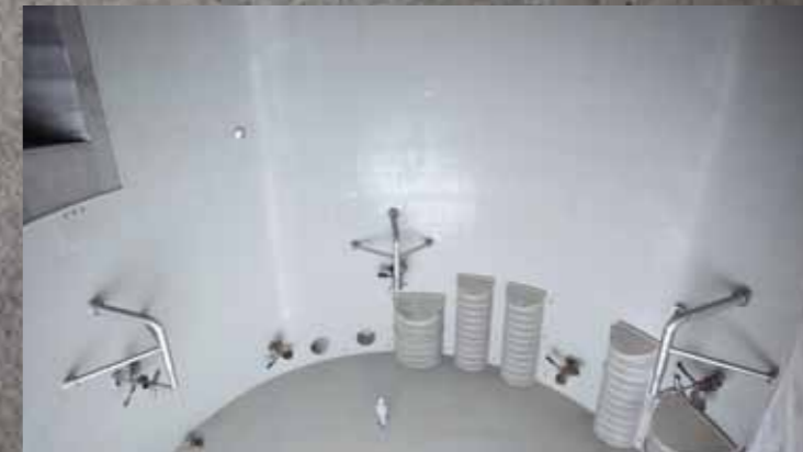
Above picture: Internal view of sump area in a flue gas scrubber built using concrete and BEKAPLAST™ including fixtures.
