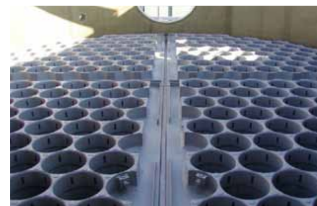
Above picture: Built-in tube bundle in a wet electrostatic filter construction.
