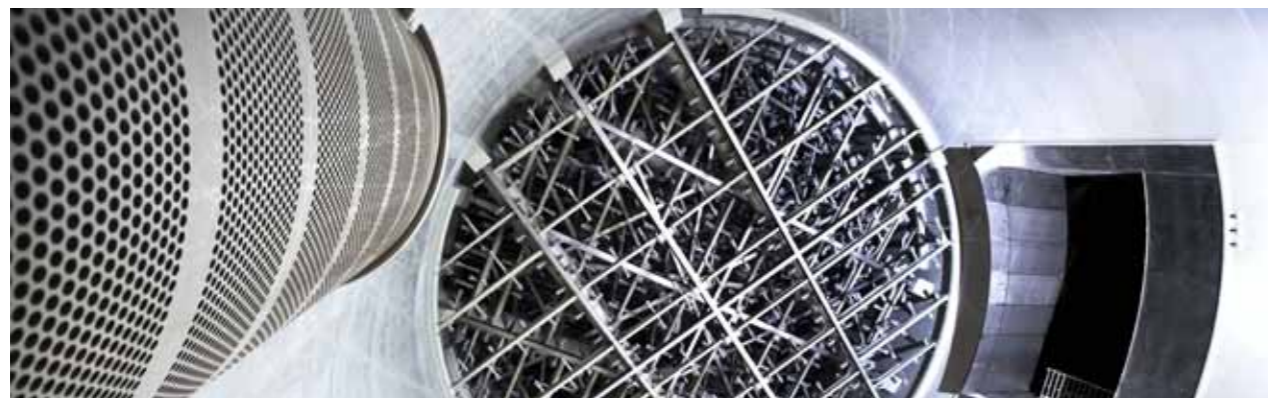
Above picture: Nozzle arrays and linings made of polypropylene in concrete flue gas scrubber.
